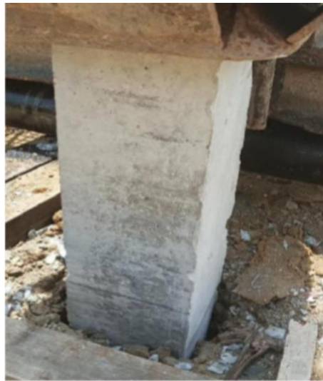
Figure 1. Precast reinforced concrete minipile 200 mm × 200 mm (Source: Project documentation, Mahakam West Park Residential Development, Pekanbaru)
